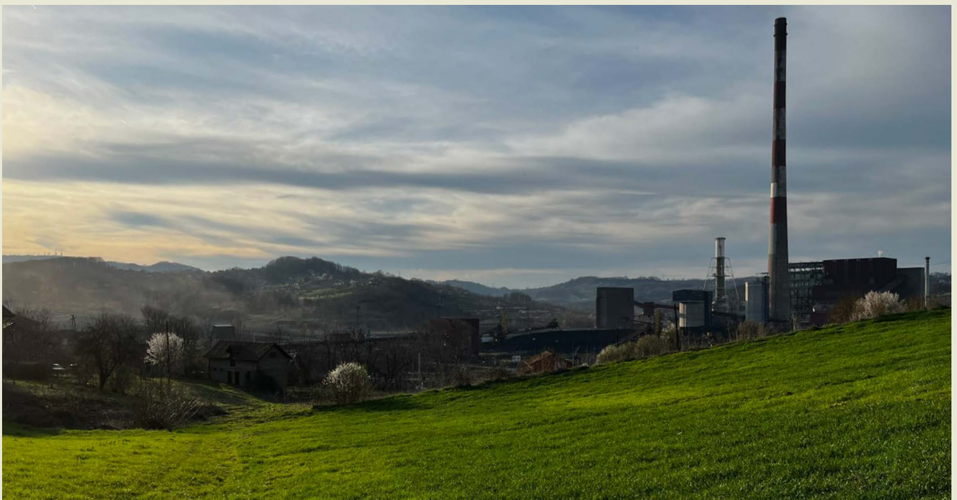
Ugljevik thermal power plant | Credit: CZZS, Bosnia and Herzegovina
